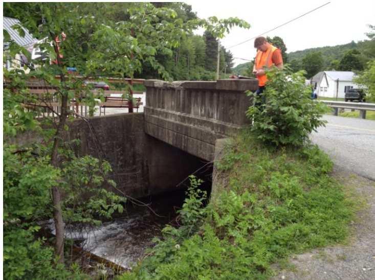
Existing Bridge 5, Looking Southeast
