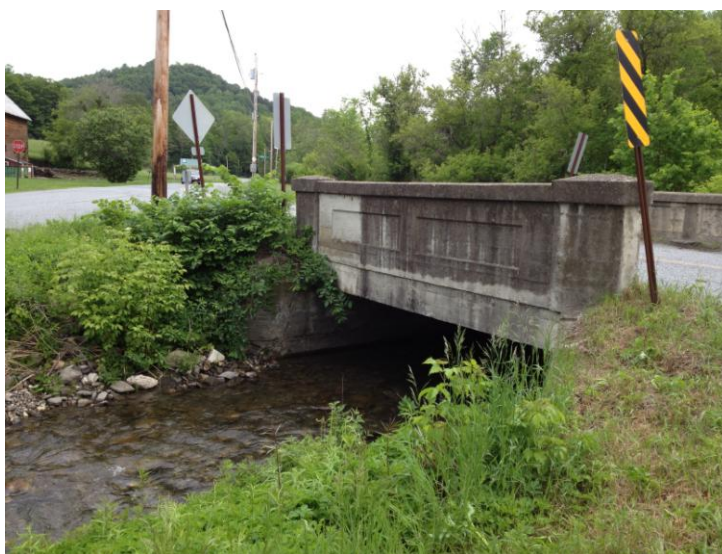
Existing Bridge 9, Looking North
