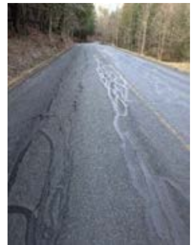
Crack sealing on Pomfret Rd
