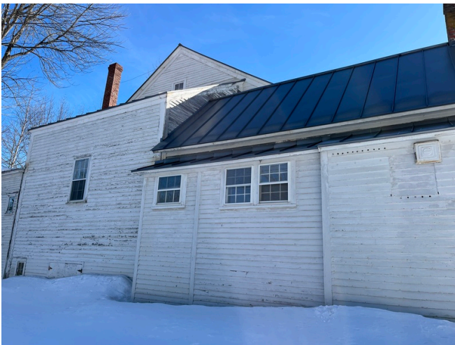
Building Exterior South Elevation
