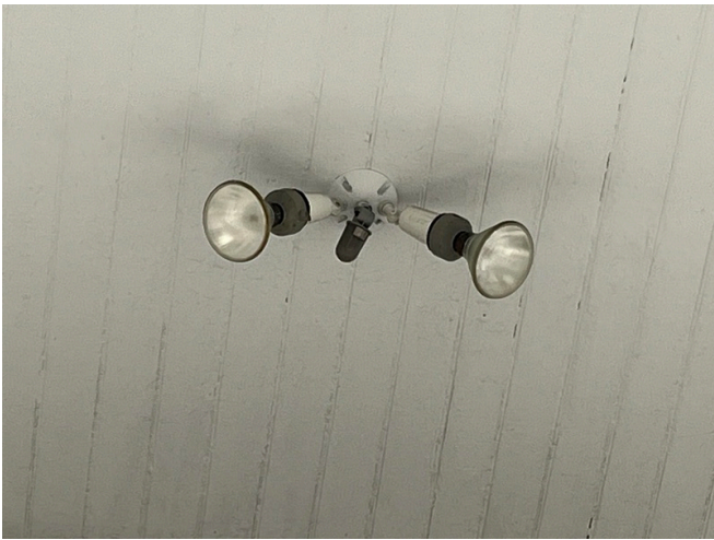
Typical Exterior Ceiling-Mount Fixture
