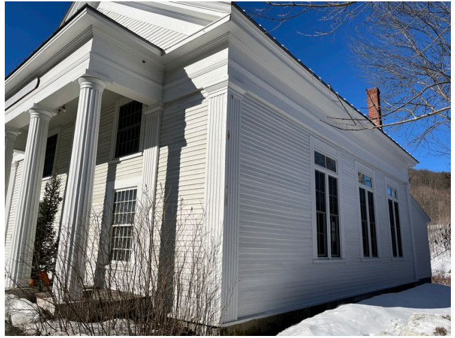
Building Exterior Northeast Elevation
