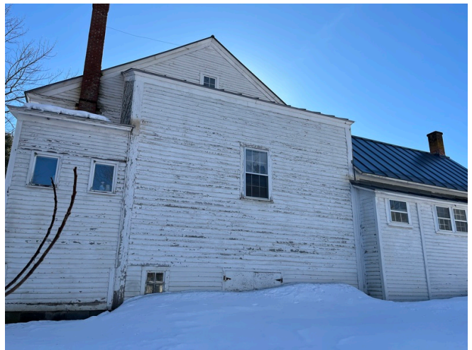
Building Exterior South Elevation
