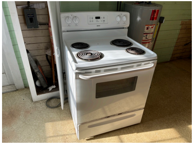
Kitchen Electric Range
