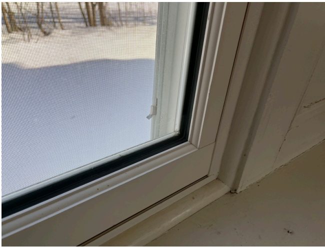
Kitchen Window Framing
