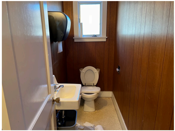
Typical Restroom Overview
