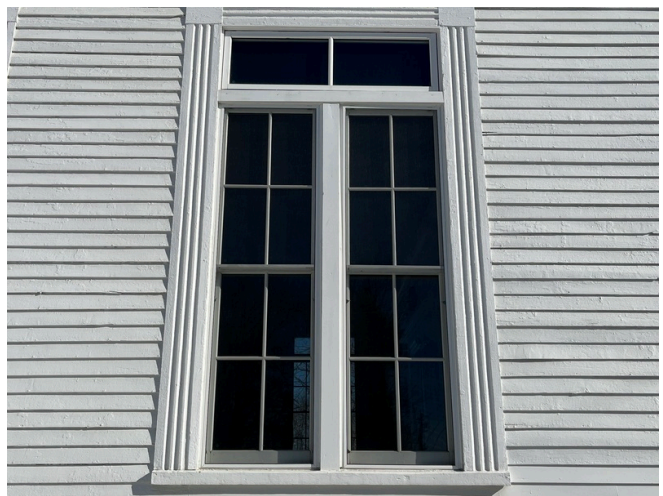
Typical Main Hall Window
