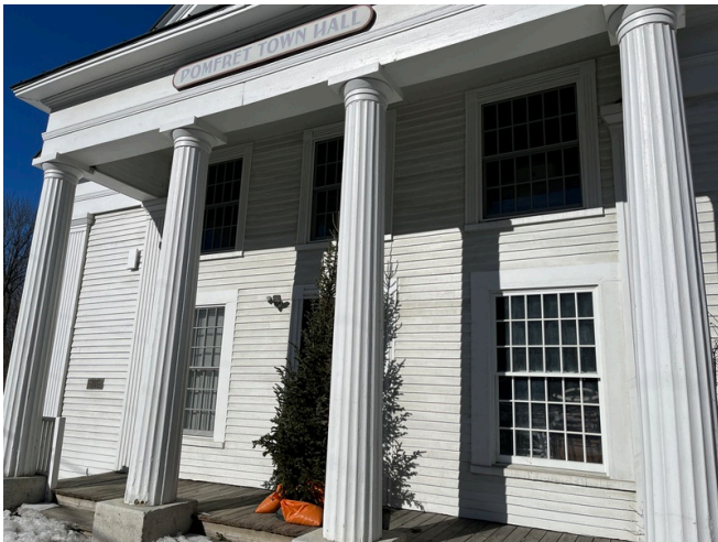
Building Exterior Entrance
