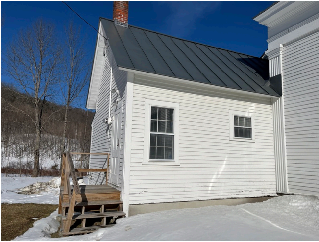
Building Exterior (Kitchen)
