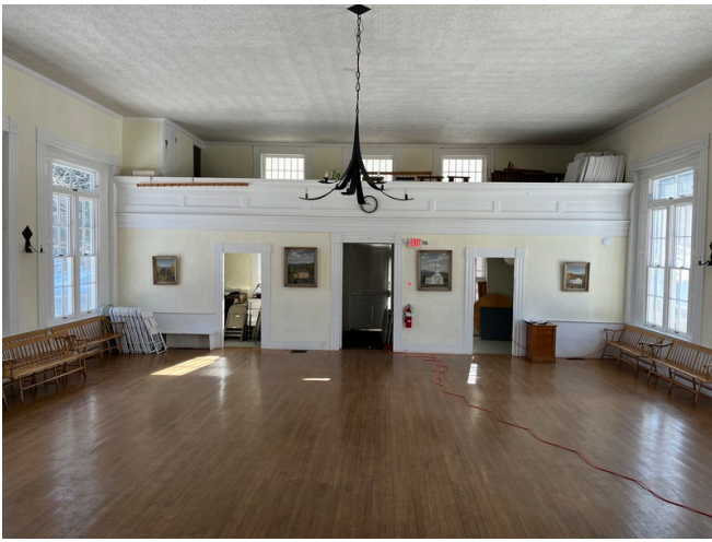
Main Hall Overview
