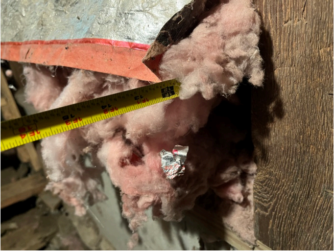
Basement Wall Insulation
