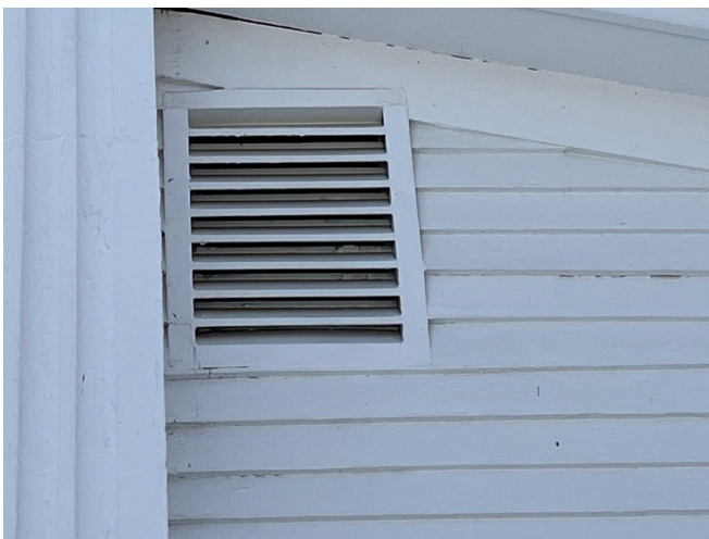
Building Gable Ventilation
