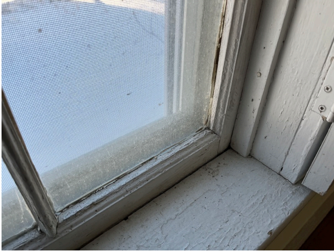
Main Hall Window Frame
