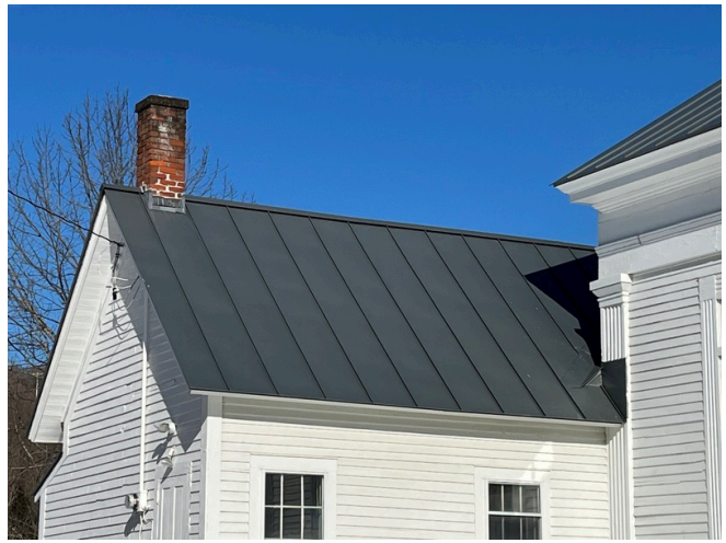
Typical Corrugated Metal Roofing
