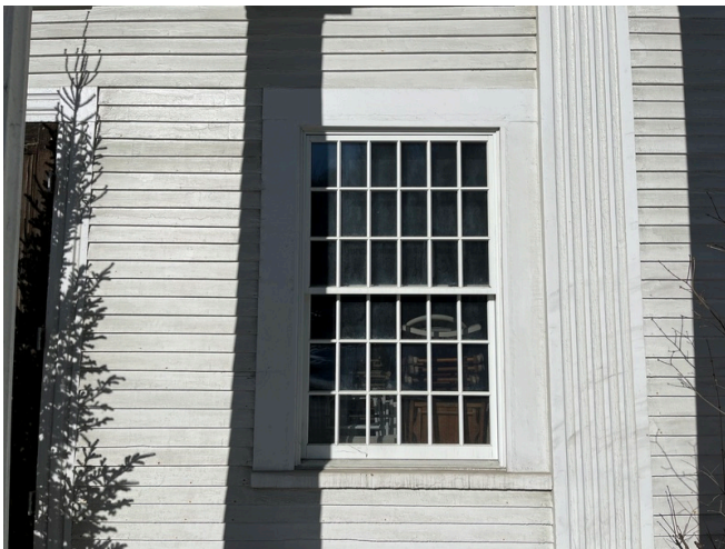
Typical Storage Room Window
