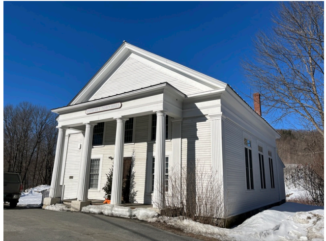
Building Exterior Northeast Elevation
