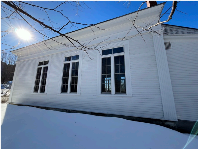
Building Exterior East Elevation
