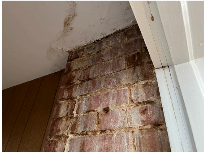
Chimney Deterioration
