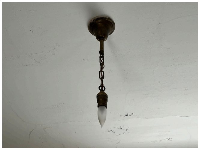
Typical Storage Room Fixture
