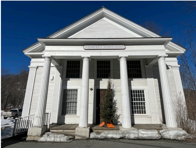
Building Exterior North Elevation
