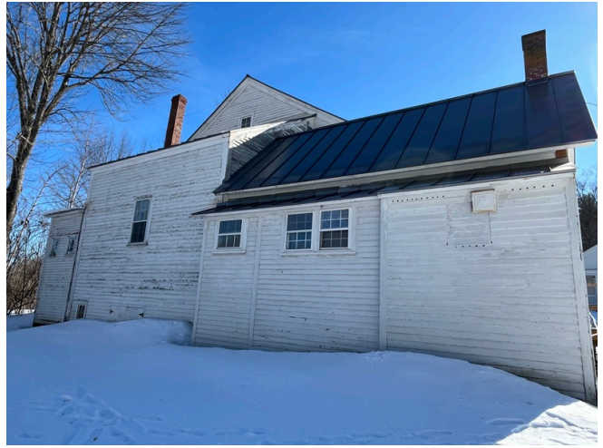
Building Exterior South Elevation
