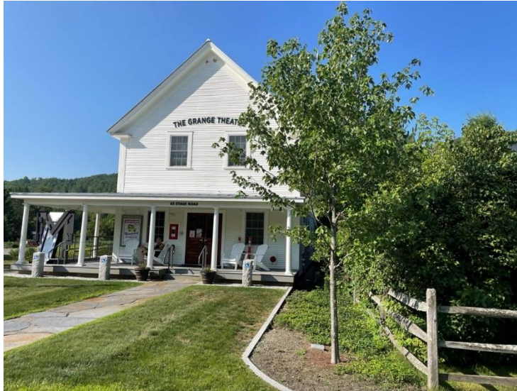
Figure 13: The Grange Theatre
