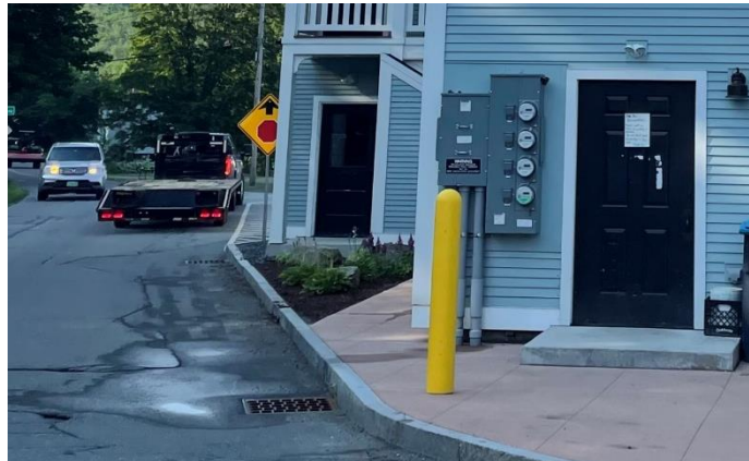
Figure 5: Drainage Grates on Pomfret Road
