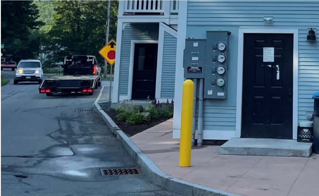
Figure 5: Drainage Grates on Pomfret Road
