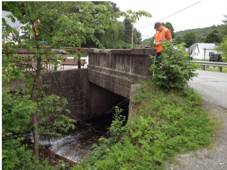
Existing Bridge 5, Looking Southeast
