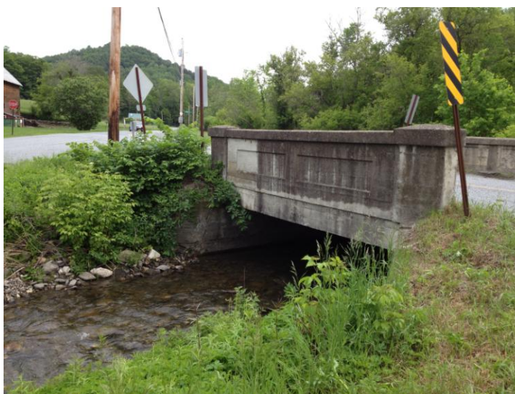
Existing Bridge 9, Looking North
