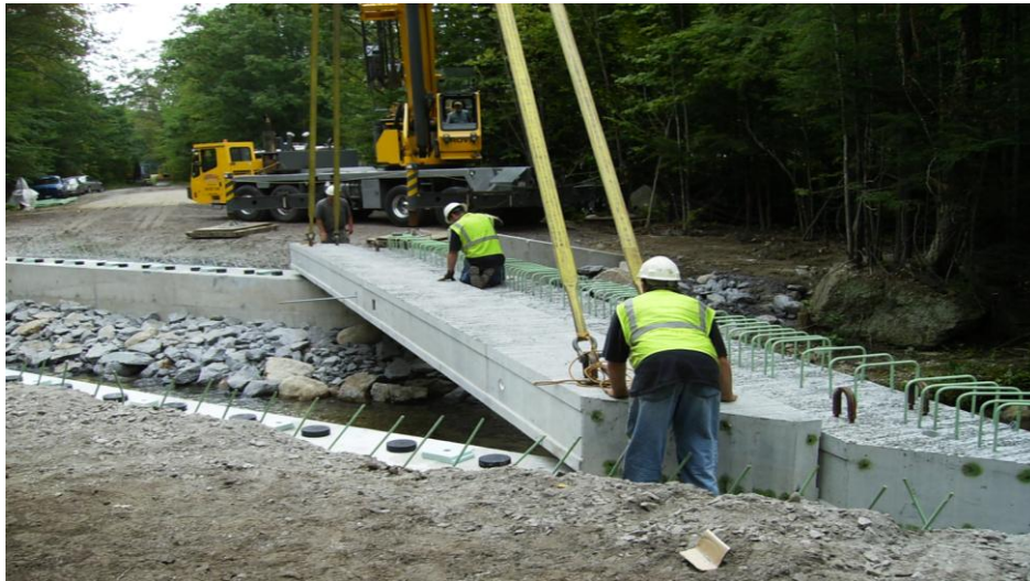
Precast Concrete Voids Slabs
