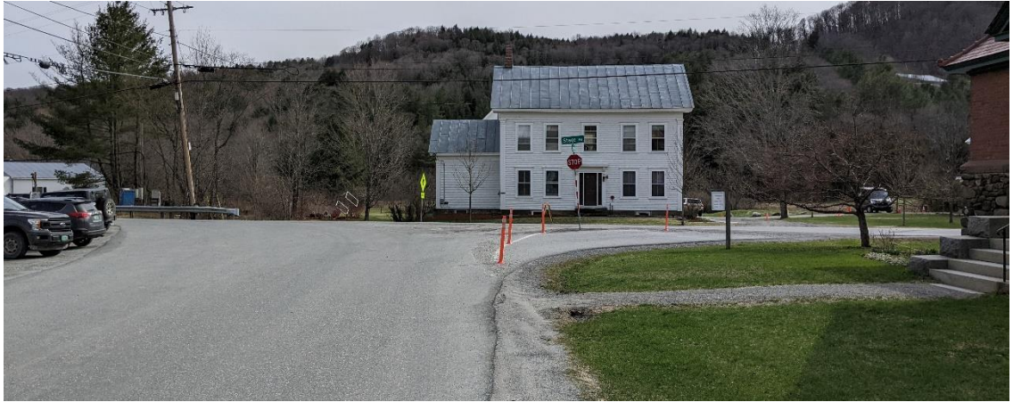
Delineators to slow turning traffic on Library Road at Pomfret Road
