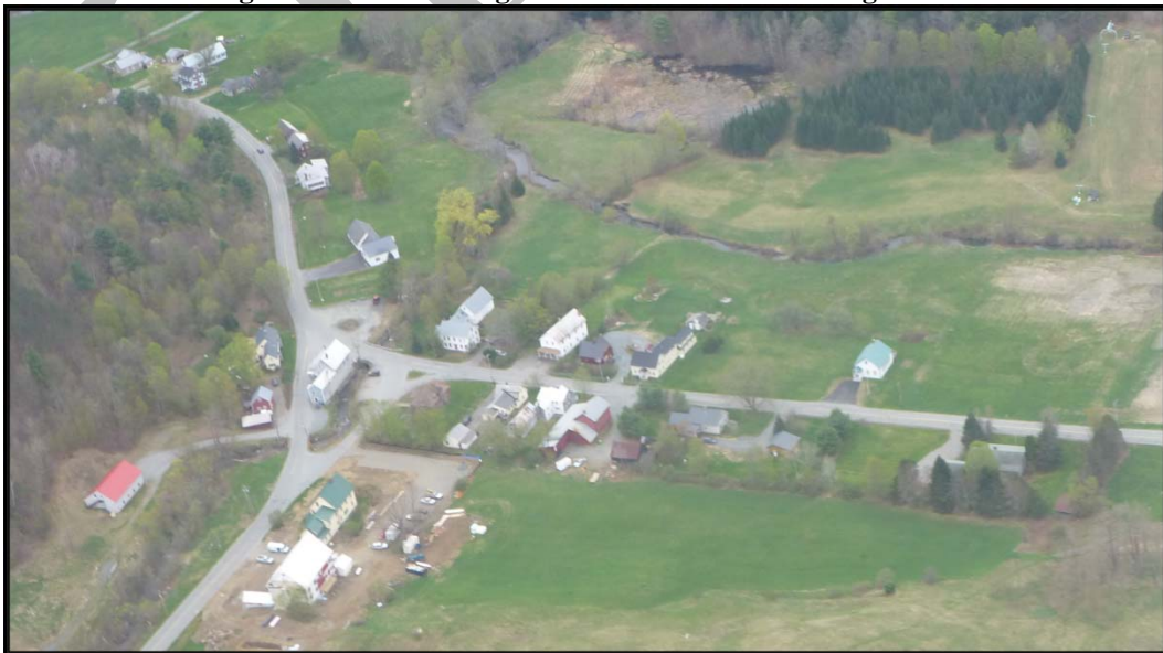
Figure 12 - Aerial Image of the South Pomfret Village Area
