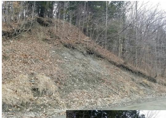
River Road bank that is failing. Goes up 50 ft in elevation. 75 feet of the bank needs to be stabilized vertically.
