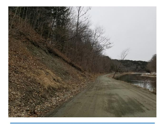
130 feet of the bank along River Road needs to be stabilized. Town of Pomfret has to re-ditch this area several times a year because of falling debris.
