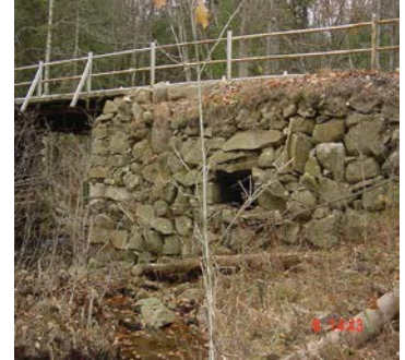
Stone Box Culvert
